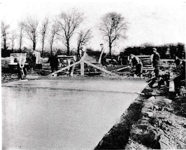
Concrete Road Construction
